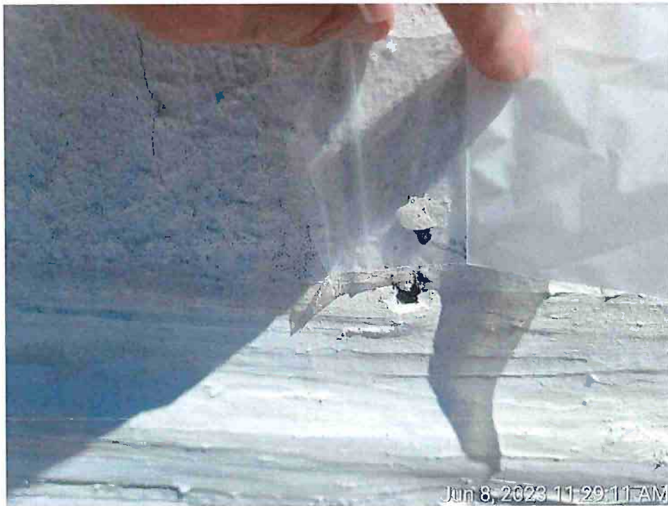
4. View of a Roof Flashing Mastic Sample
