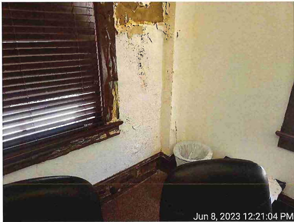
12. View of the Plaster Wall sampled in Room 101
