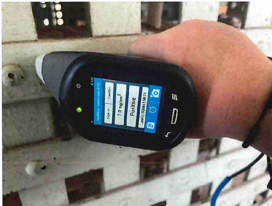
18. View of the white metal jail cells tested and positive for Lead – Based Paint
