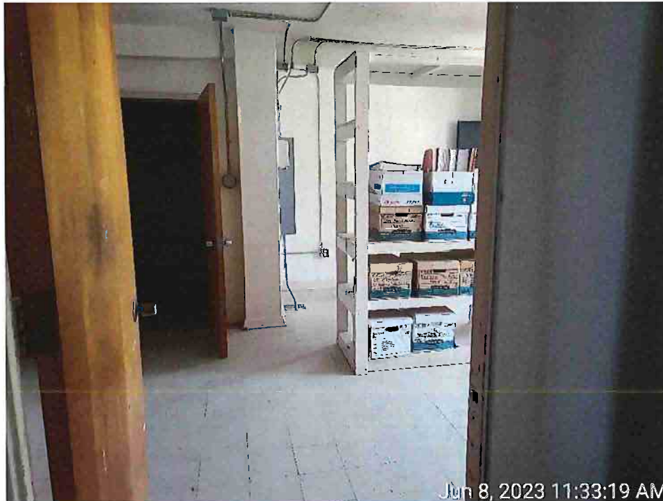
6. View of the 3 rd Floor Records Room
