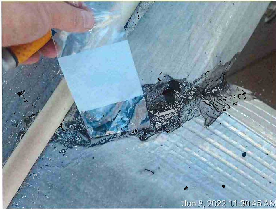
5. View of a Rolled Asphalt Roof Mastic Sample
