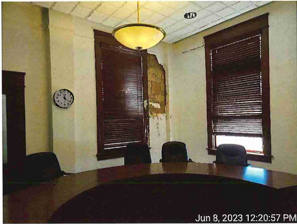
11. View of the Plaster Wall sampled in Room 101
