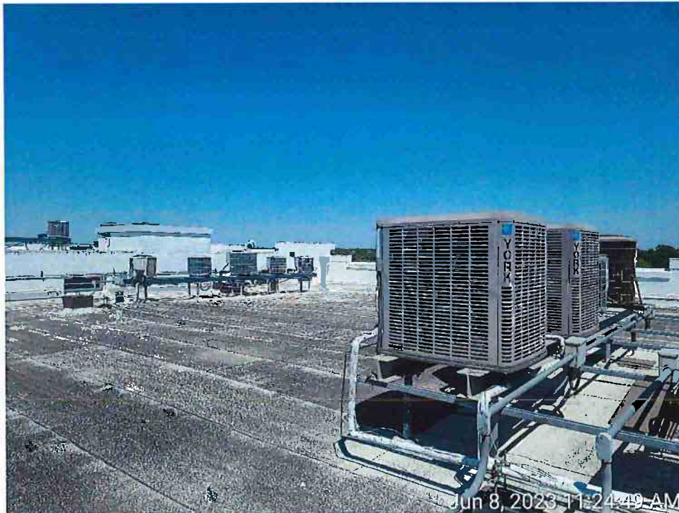
2. View of the Roof of Live Oak Courthouse
